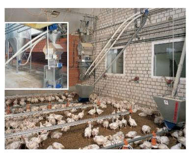
Supplementary wheat feeding can be a good alternative in growing broilers for saving feed costs and for improving the birds' health. The technical requirements for this are a second silo, the FW 99-B feed weigher, conveying augers (FlexVey) from the silo to the weigher and to the feeder as well as the ViperTouch production computer.
