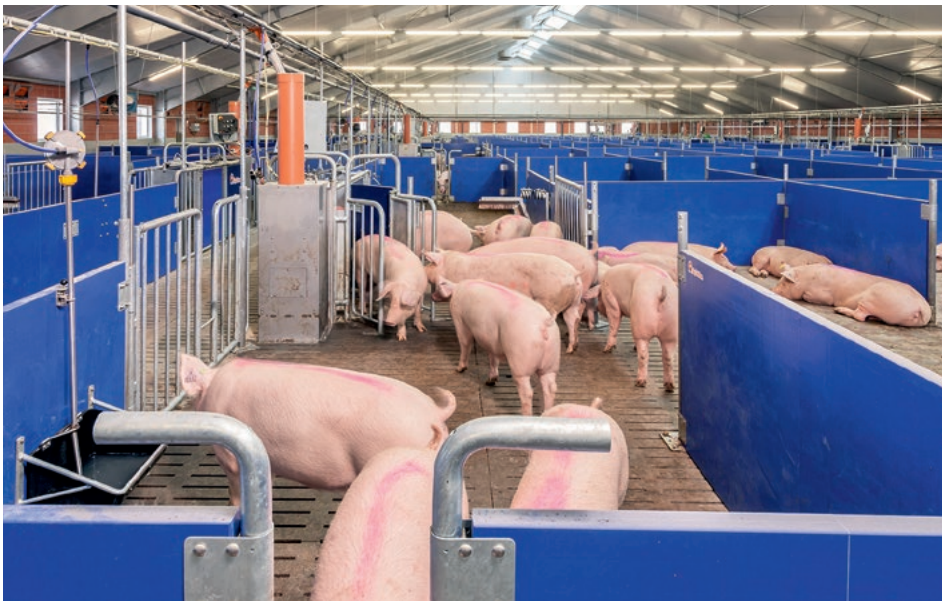
View of a waiting area equipped with the computer-controlled ESF station Call-Inn pro
