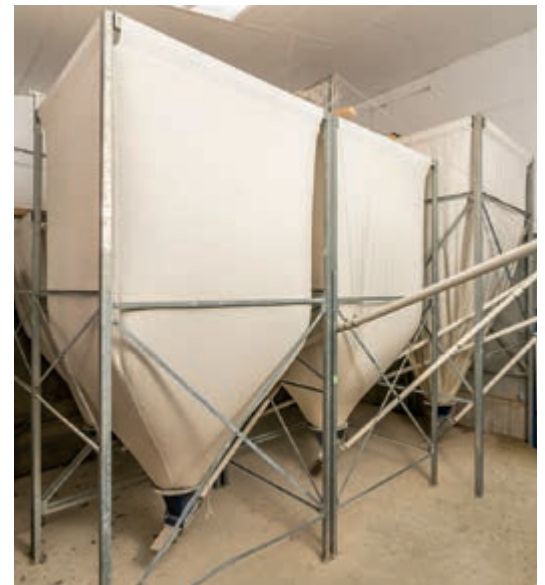
Inside silos made of Trevira fabric
