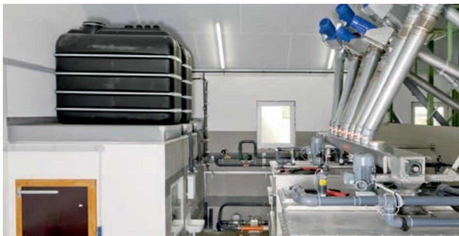
Feed kitchen with 2-tank residue-free feeding system and two 2000 L fresh water tanks
