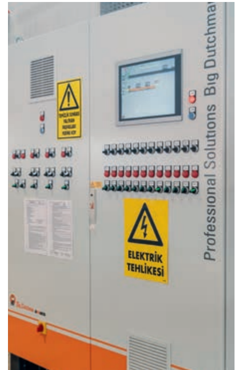
Control cabinet with 15" touch display for control of the egg flow towards the packer
